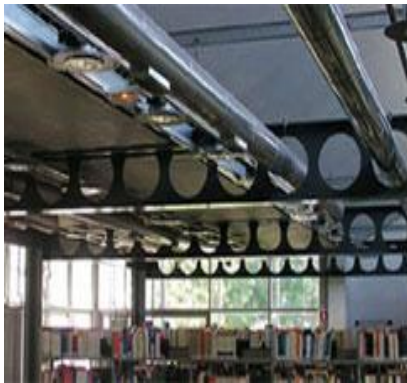
Figure 5.3: Example castellated beams coordination with distribution systems from ArcelorMittal
